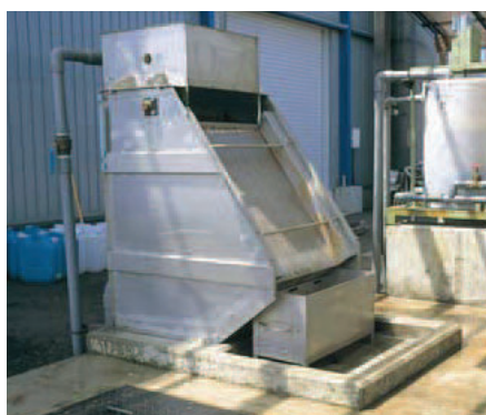
Site: Dairy products plant
